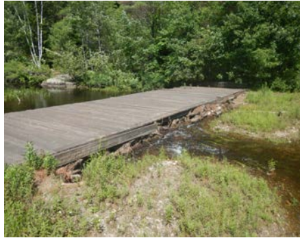
Hammond Pond Dam
